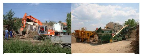
Photo2: Demolition of private homes in Kosovo with loading of the debris to be transported to the nearby recycling depot. Source: Golder Associates. Photo 3: Crushing and screening of the debris for use as road based material in the rehabilitation of war damaged roads. Source: Golder Associates.
