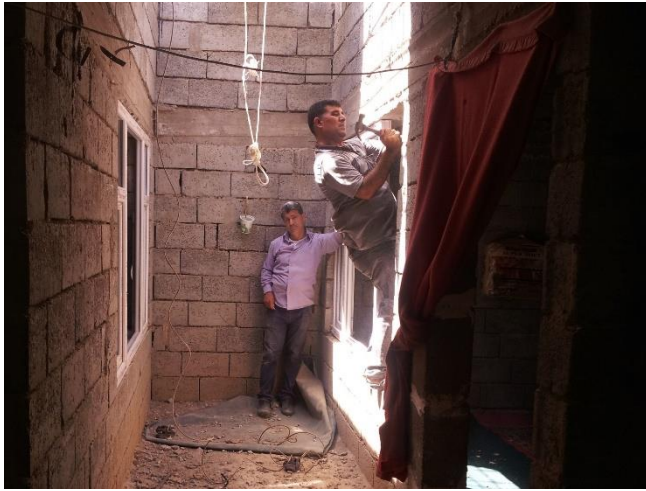
Carpenter repairing a shelter in Kirkuk
