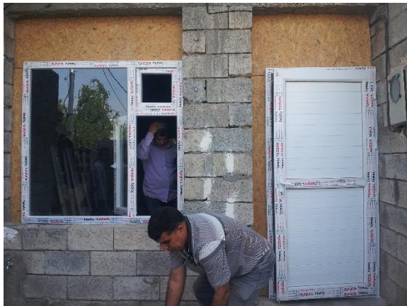
Newly installed window and door, Kirkuk
