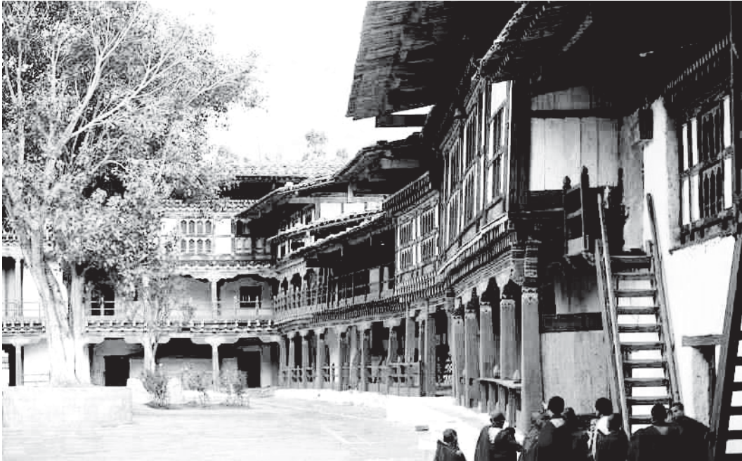
Inner court yard of Wangdue Phodrang Dzong. Heavy use of wood in the construction of traditional buildings make them highly susceptible to fire hazards. (KD)
