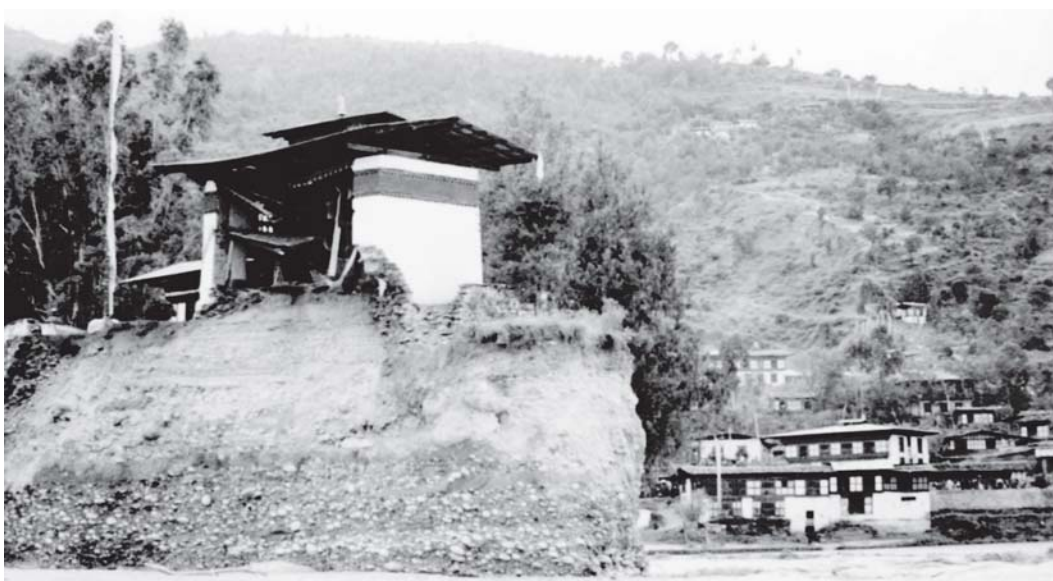
Impact of 1994 flood on one of the oldest temples in front of Punakha Dzong
