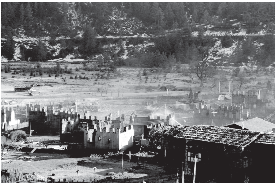
25 traditional houses in Yangthang village in Haa were completely burnt down by fire in 2002.
