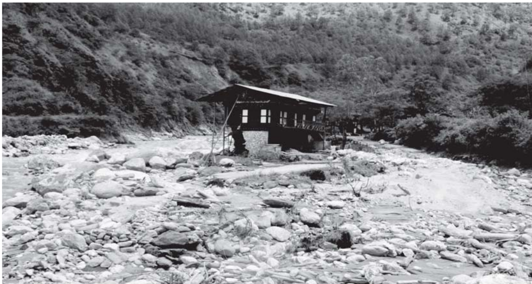
A partially damaged house in Lungtenzampa, Trashigang after the 2004 monsoon flood (Kuensel)
