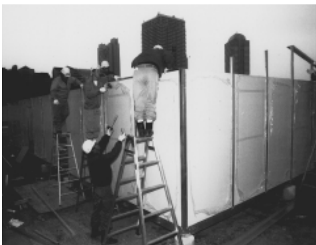
Temporary housing under construction
