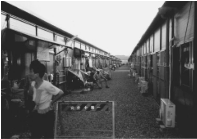
Temporary housing site, Kobe
