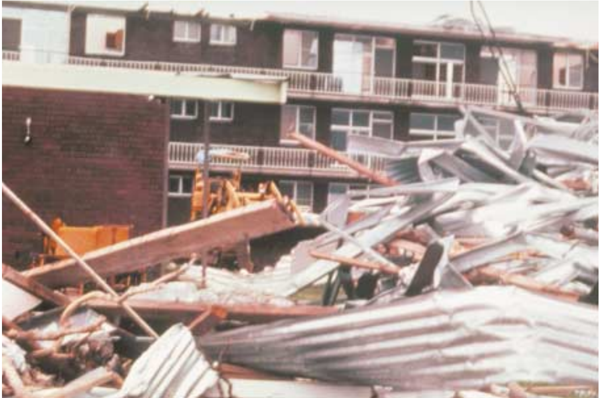
Structural inadequacy is exposed by failure of so many buildings. Compare for instance the building in the rear to the building in the foreground
