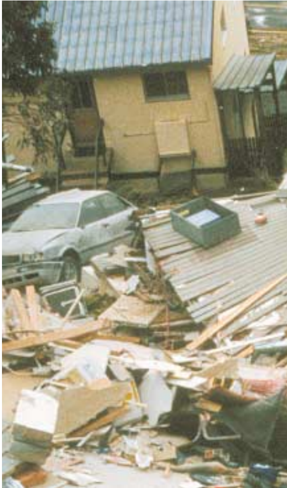
There are many buildings older than thirty years that should not fail to the extent they do
